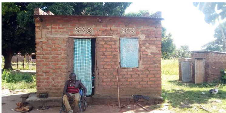
Photo showing Mr. James in front of his one iron roofed house after completion.
