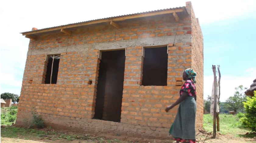
A Photo showing the house being constructed by Ms. Bayoa Celina.
